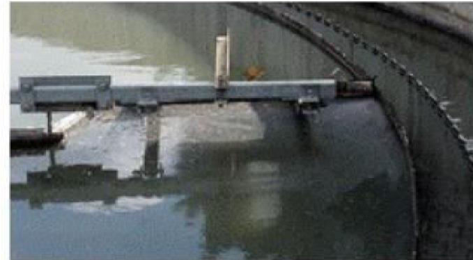
Revolving bar to collect and remove floating scum.
