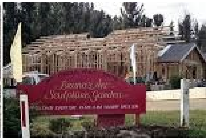
Buildings rebuilding in Marysville, Australia
