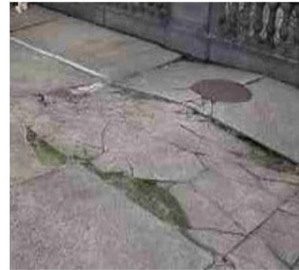
Fig. 4: Frost Heave damaged Concrete
