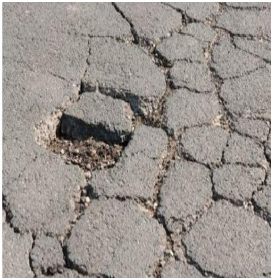
Fig. 5: Pavements Cracks due to Frost Heave
