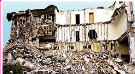
STRUCTURAL COLLAPSE (Building collapse)
