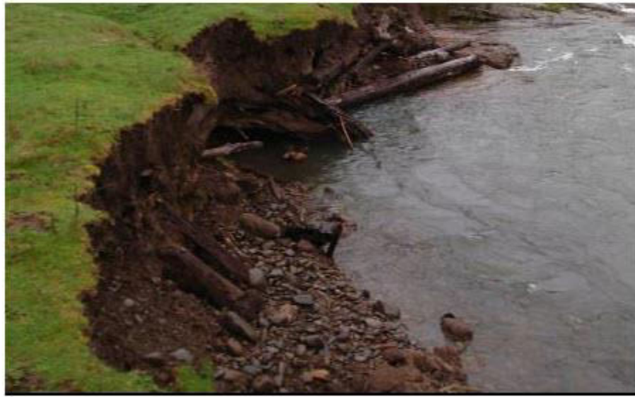
Fig. 3.5. Stream bank erosion. (Source: www.sswc.org )
