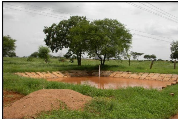
Fig. 15.2 Farm Pond Lined with Kadapa Slabs
