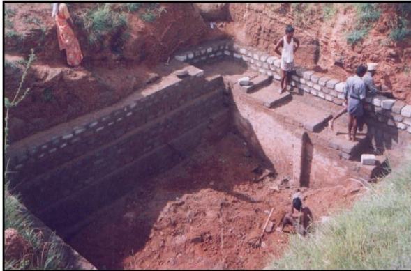
Fig .15.3 Farm Pond lined with Cement Bricks
