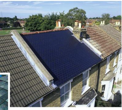
Panels of solar Solar shingles cells
