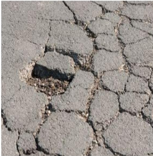
Fig. 5: Pavements Cracks due to Frost Heave
