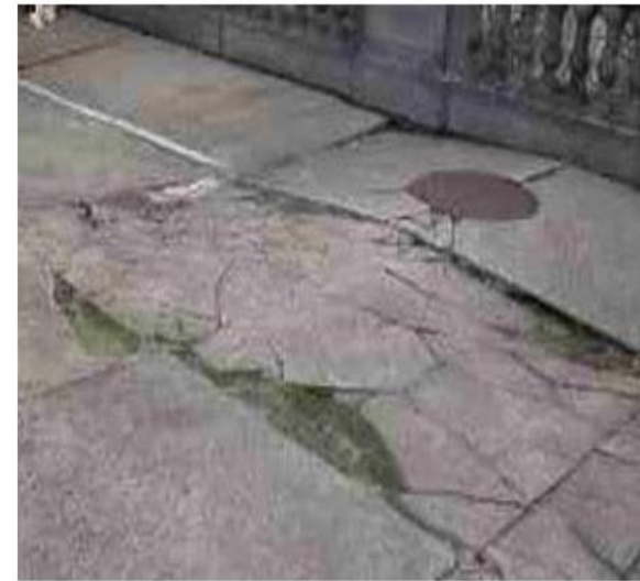
Fig. 4: Frost Heave damaged Concrete
