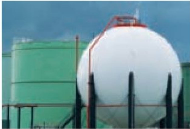
Thin-walled spherical pressure vessel used for storage of propane in this oil refinery
